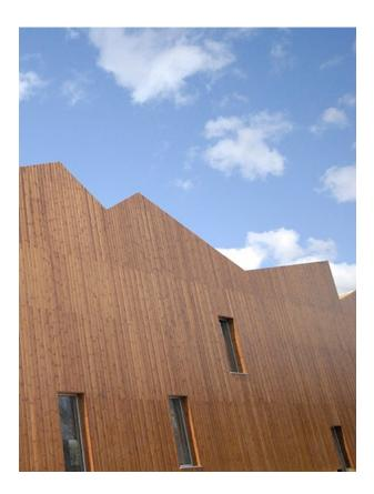
Finnish Lunawood Thermowood is a beautiful wood material produced using natural methods, heat and steam. Thermowood is dimensionally stable, resistant to decay and non toxic. It can be used for interior and exterior applications. Lunawood is an eco-friendly natural product, which is easy to machine and install.
