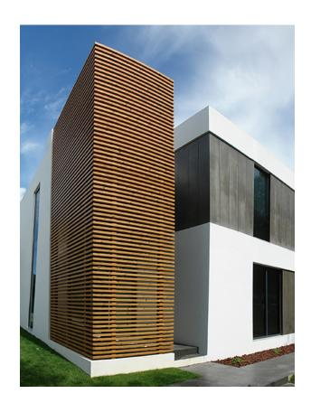
Finnish Lunawood Thermowood is a beautiful wood material produced using natural methods, heat and steam. Thermowood is dimensionally stable, resistant to decay and non toxic. It can be used for interior and exterior applications. Lunawood is an eco-friendly natural product, which is easy to machine and install.
